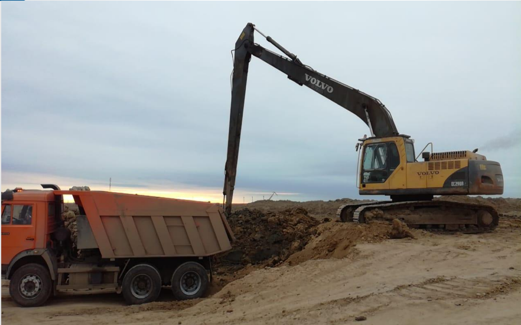
Excavator VOLVO EC 290 , boom 20 м., power performance 28 м3
