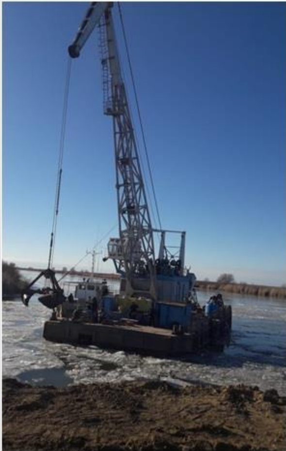
Crane boat PKL-412
